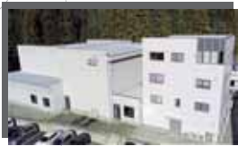
Main Office Nagano EMC Center
